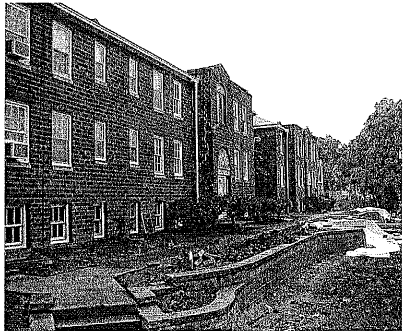
New sidewalks and a stone retaining wall are but a few of the improvements that Larry had made to the property. He plans to landscape the grounds around the apartments and install a fence around the entire complex. Although the project has not been completed yet, it has already improved the appearance of the entire area. Drive by and see this "new" addition to the neighborhood! (Photos by Terry Wilwerding)
